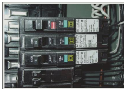
Example of AFCI circuits in panel
