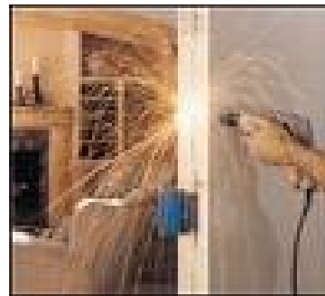
Drilling hidden wires
