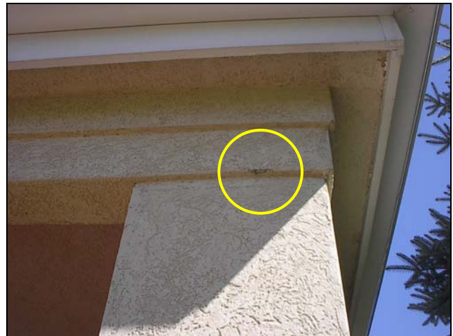
Damaged stucco requires repair per manufacturer detail
