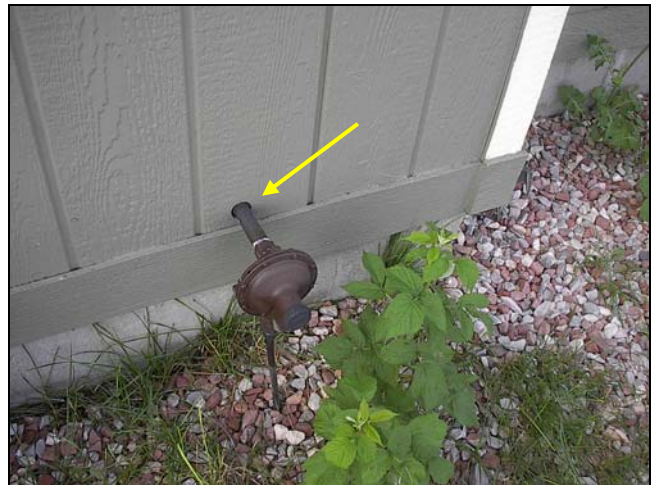
All penetrations require sealing
