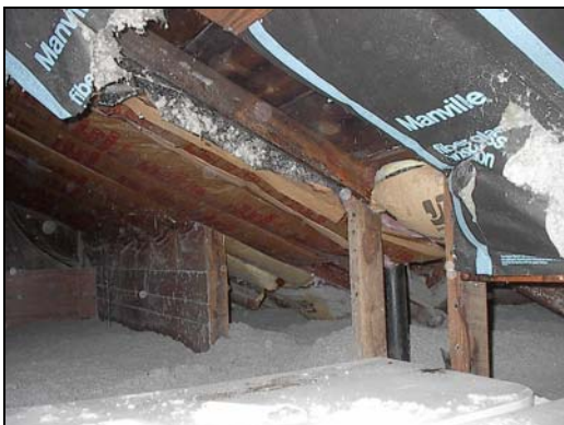
Restricted access in attic
