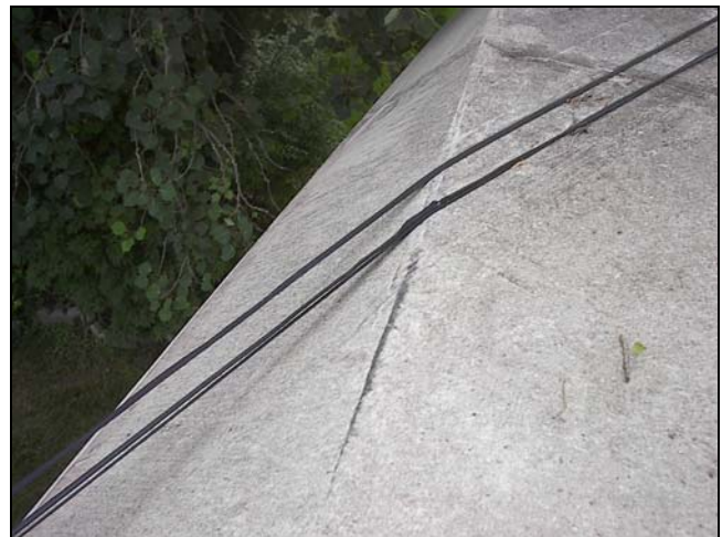
Failure may result due to mechanical abrasion
