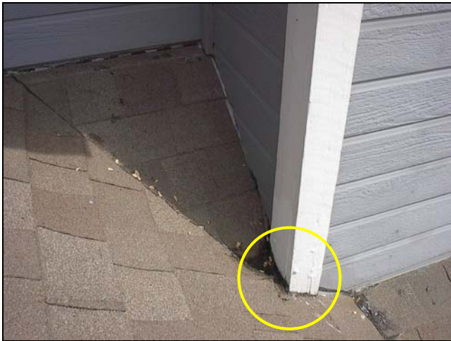
Wood trim at short valley above garage
