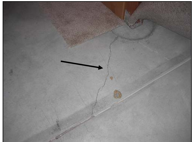
Cracking evident in the concrete slab floor
