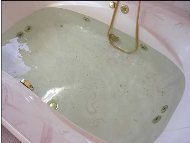
Debris in jetted tub
