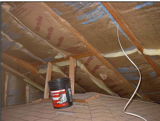
Unconventional supports attached to original roof
