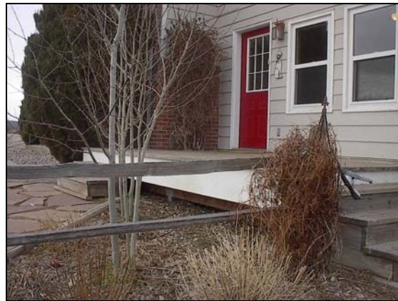
Height of deck floor is approx. 26-inches above grade
