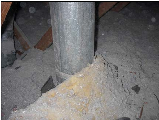
Paper backed batt lying against chimney vent
