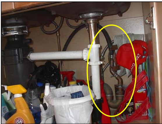
Drain connection for dishwasher
