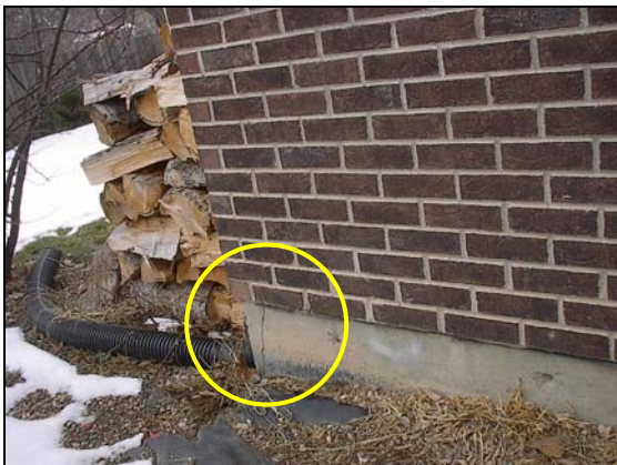
Inconsequential crack in foundation wall
