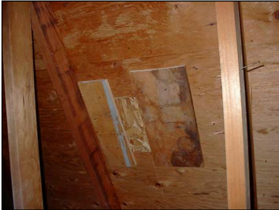
Repair to sheathing
