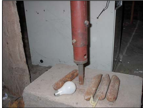
Supporting pins of telescoping column
