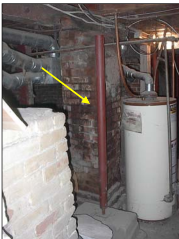
Telescoping (temporary) column
