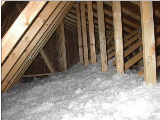
Adequate levels of insulation
