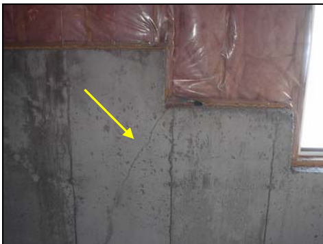
Crack in foundation's west wall
