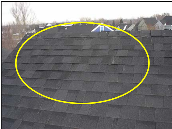
Section of roof cover that apparently was replaced
