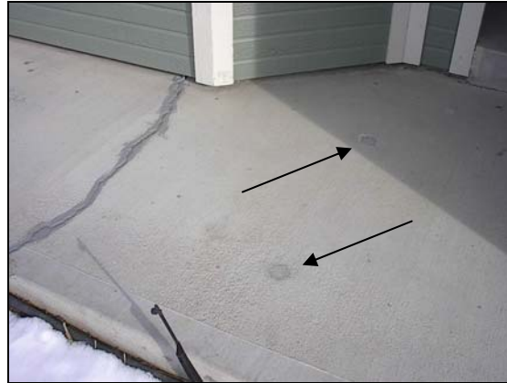
Evidence of mud-jacking repair
