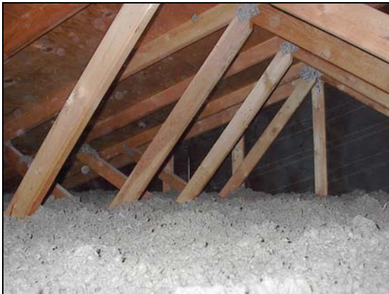
Adequate levels for insulation
