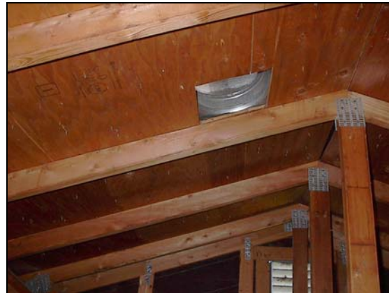
No evidence of water penetration
