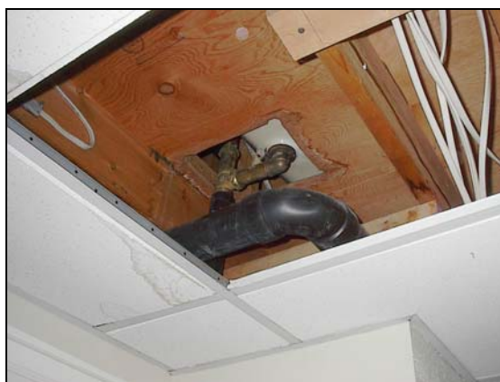
Further investigation revealed dry subfloor
