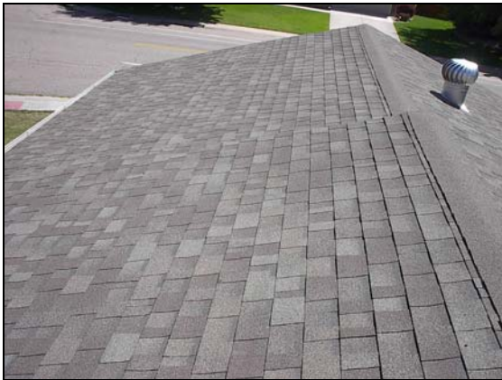
Newer roof is in satisfactory condition
