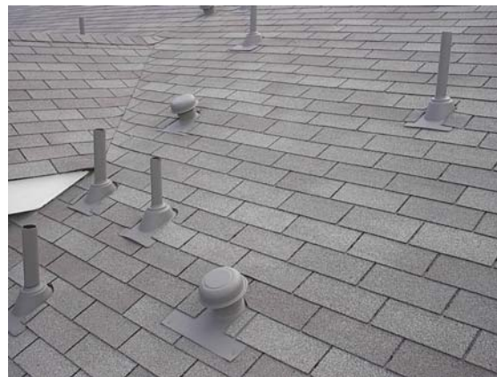
Overall, the roof is in satisfactory condition
