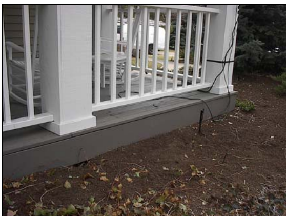
Inaccessible front porch deck
